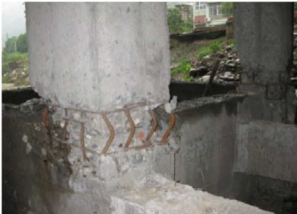
Frame damage at the bottom of a column
