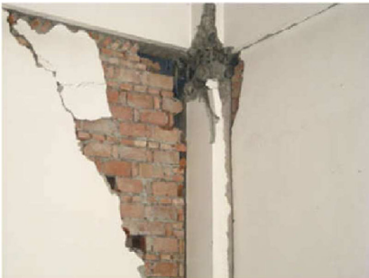
Frame damage at the top of a column
