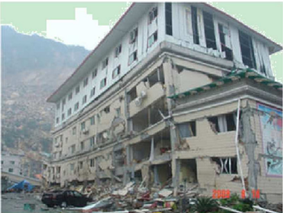
Collapse of the first floor in a frame structure
