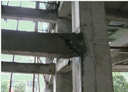
Damage of frame structure in beam
